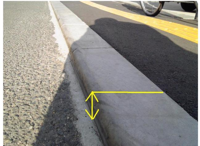
Figure 1: Sharp drop in the road level
